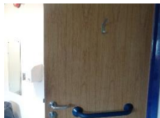
The coat hook is too high for a person in a wheelchair.
